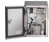
Emerson offers turnkey solutions of best-in-class ASCO and AVENTICS products mounted in stainless steel integrated enclosures. Components can include directional and fluid control valves, G3 fieldbus electronics, and FRLs. These NEMA wash-downrated solutions eliminate contamination and protect components from corrosion that may cause downtime. They also eliminate complex tubing, routing, and bulkhead fittings.
